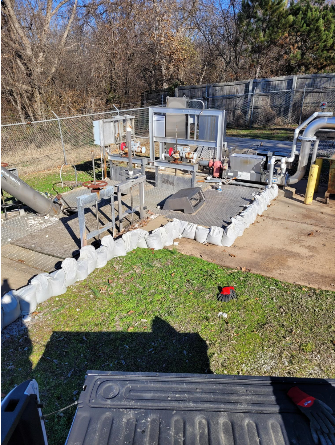
Sandbags placed around the existing headworks channels
